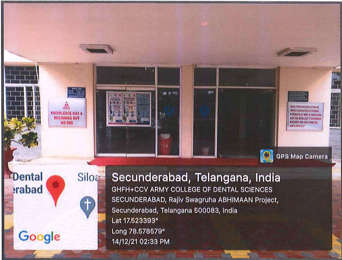
Fig-10: CCTV in college campus
