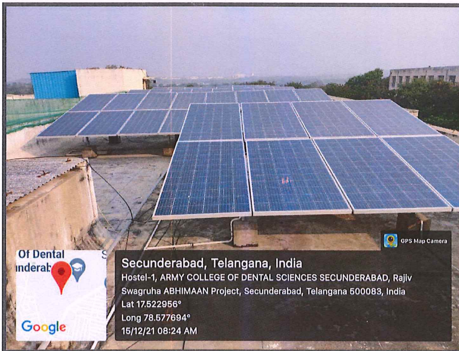
Fig-2: 25 KW solar roof top power grid
