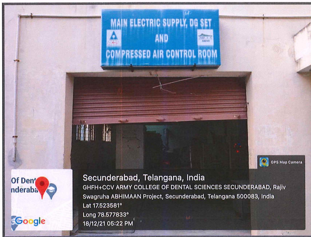
Fig-13: Main Electric Supply room
