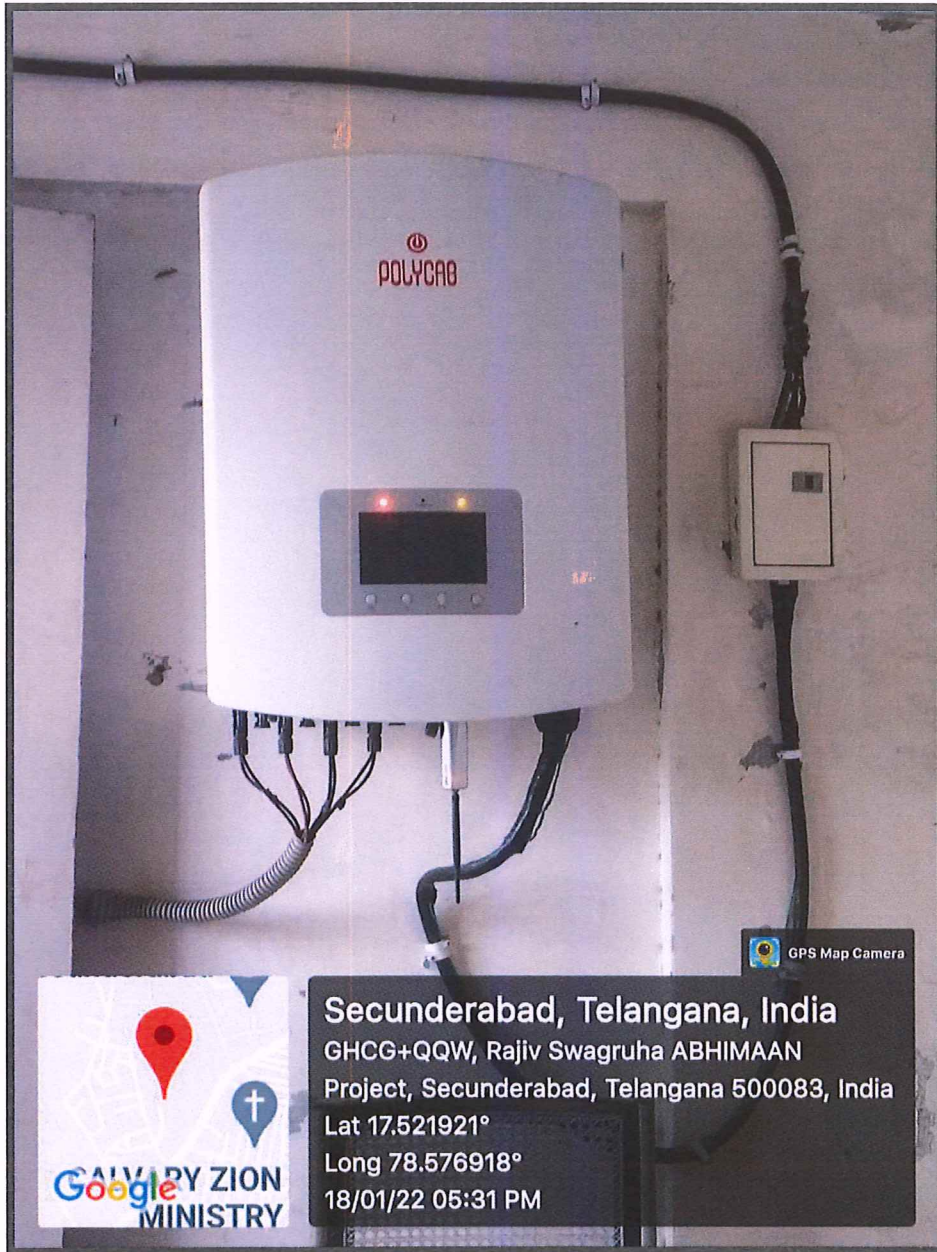
Fig-3: Polycab string grid tie inverter
