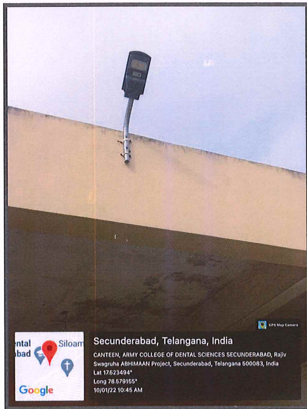
Fig-8: Solar flood light installed at MT Parking area
