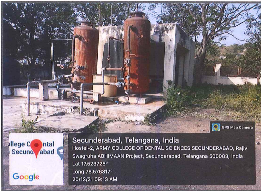
Fig-5: Water pump house
