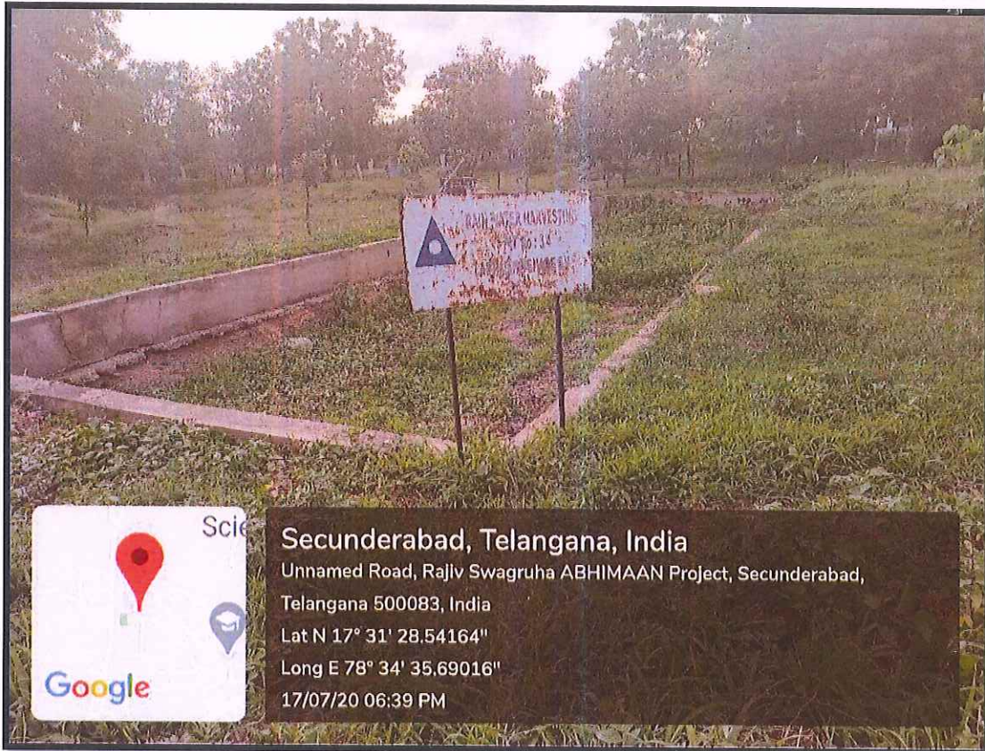
Fig-1: Rain water harvesting
