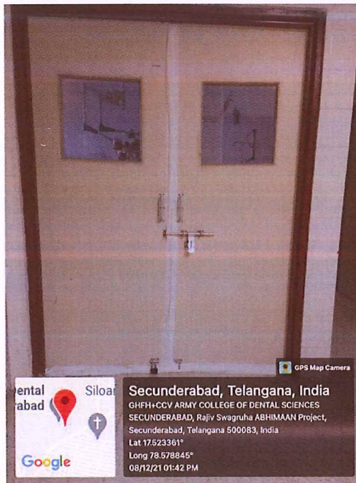
Fig 10 B Sealing of Doors for Adequate Disinfection
